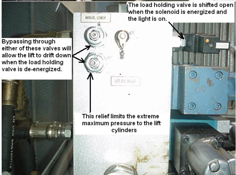
When observing the lift with the locking valve solenoid de-energized, the cylinders retracted, allowing the stacker to drift down. This meant that the problem had to be with the locking valve, the manual or relief valve, or bypassing in the cylinders. I was told that the cylinders had been recently rebuilt.
