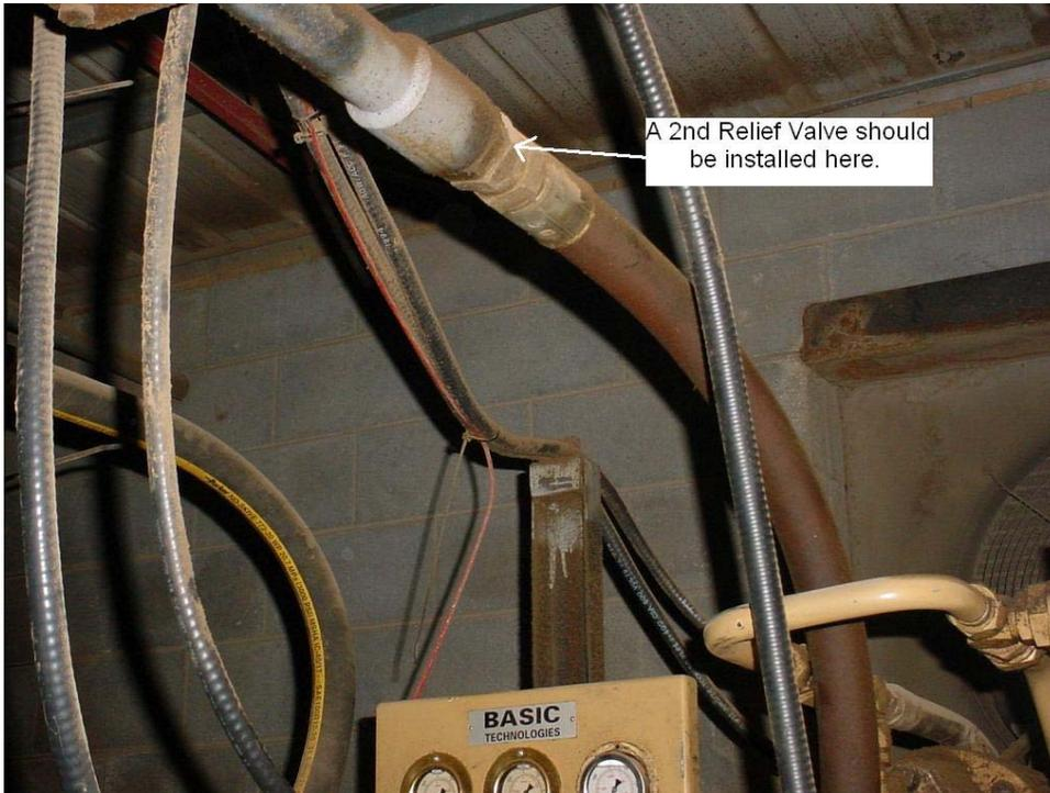
The relief valves tank lines can be connected to the reservoir here.
