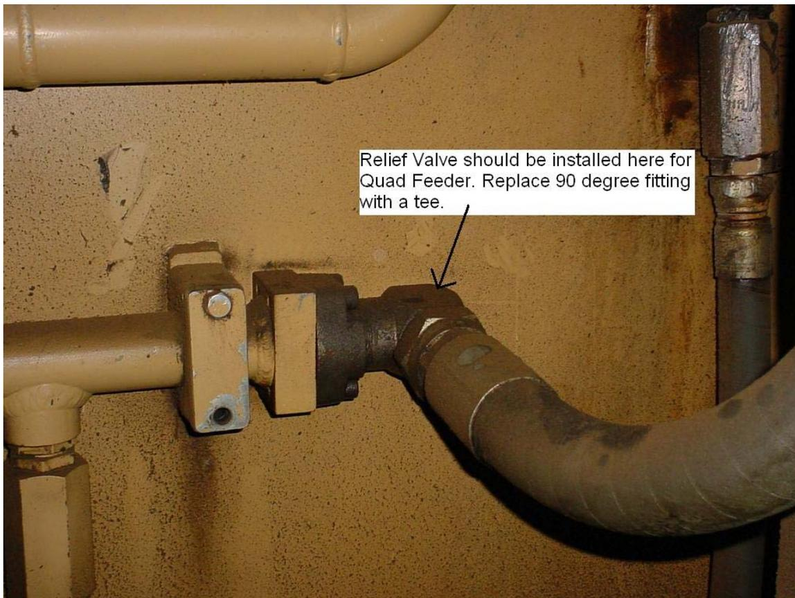
A second relief valve needs to be installed down stream of the Slasher Deck pumps.
